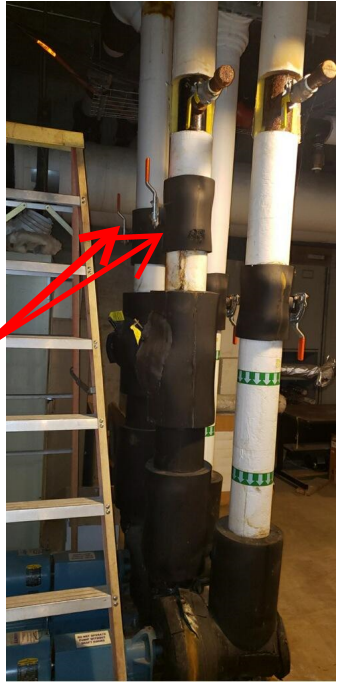
9th Open valves on discharge of pumps
